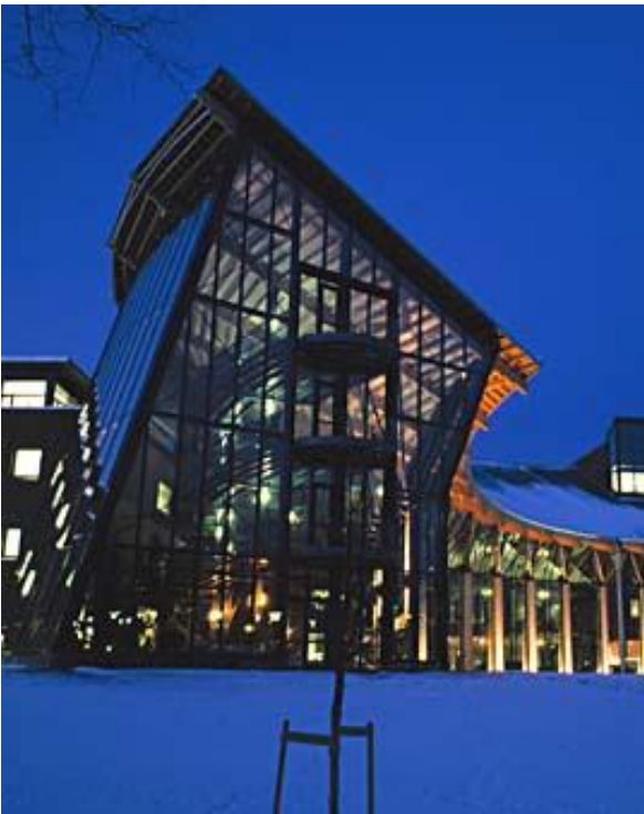
Statoil R&D Centre, Trondheim
