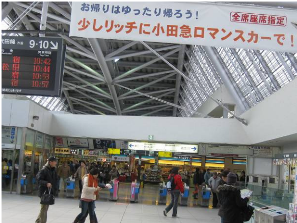
SOLAR ARRAY INTEGRAL TO ODAWARA STATION ROOF
